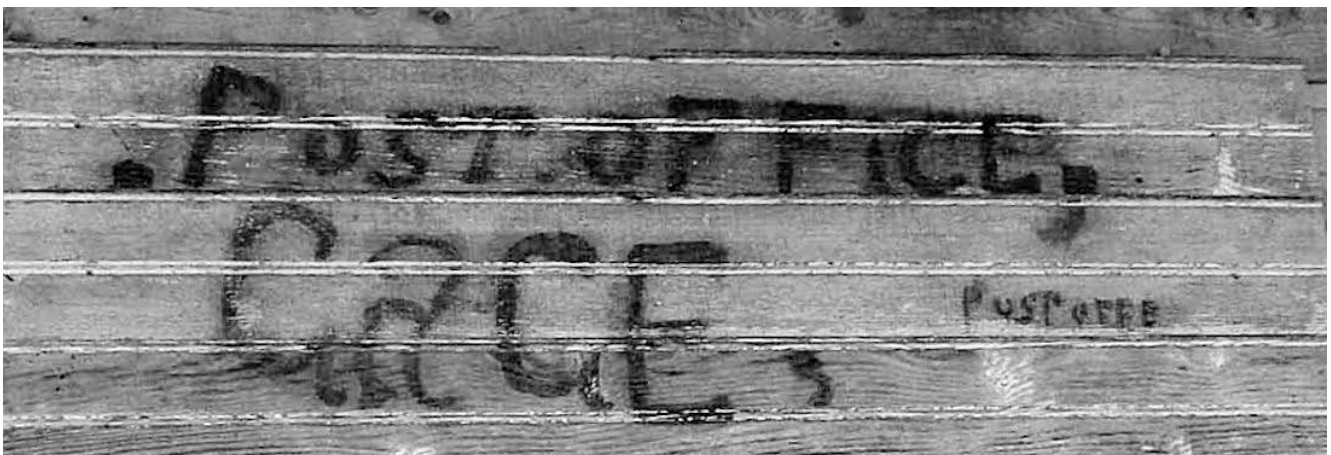
The old post office sign from the porch of the Boyd House. This was the only part of the house that had weatherboarding on it at the time.
