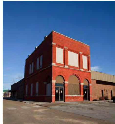
Rear: Research Library Corner: Restoration of 1904 First National Bank Building to be used as Assembly Room and Museum; Right: More Museum display area
