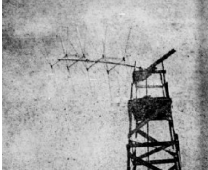
Kennerly Cunningham's aerial bent by the tornado. (Photo courtesy Grundy County Herald)
